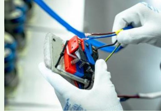
Water pump detection
